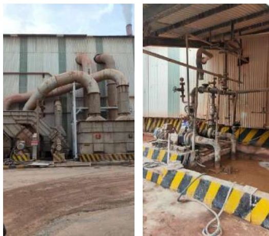
Gambar IX. 5 Sistem Scrubbing NPK Granulasi II
