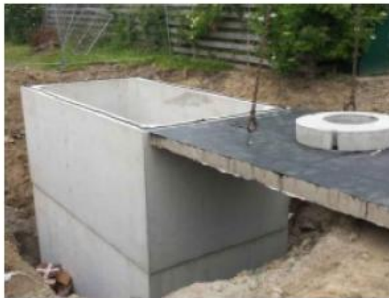
Gambar 2. 16 Reservoir Beton Cor
