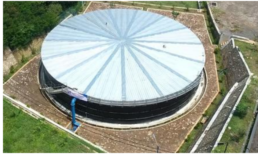
Gambar 2. 15 Reservoir Tangki Baja
