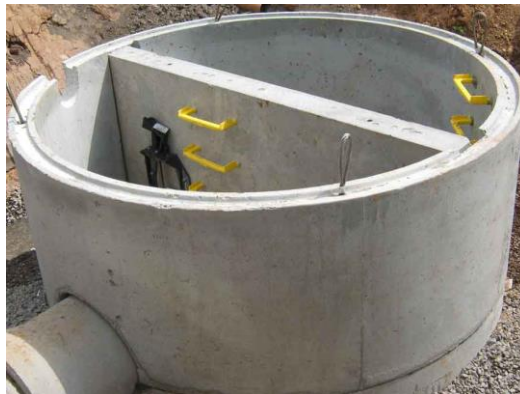
Gambar 2.23 Reservoir Beton Cor
