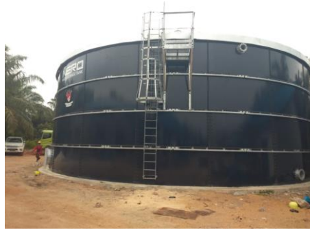
Gambar 2.22 Reservoir Tangki Baja
