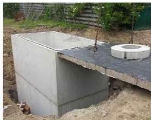
Gambar 2. 22 Reservoir Beton Cor
