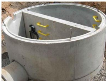
Gambar 2. Reservoir Beton Cor
