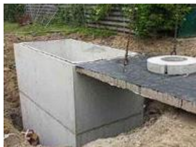
Gambar 2 . 24 reservoir beton cor
