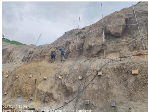
Gambar 4.7 Proses Grouting
