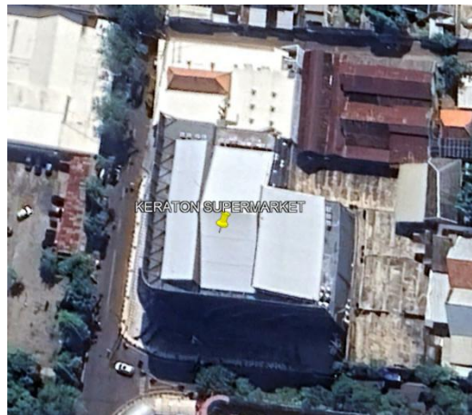
Gambar 1.4 Keraton Supermarket Sumber : Google Earth
