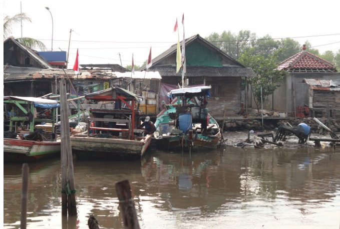
Figure 1. 2 Condition of Karangantu Port, 2025
