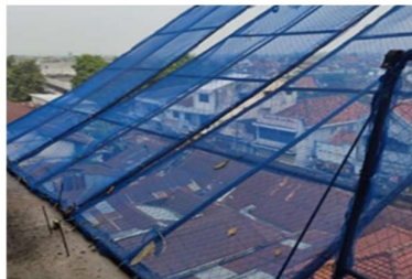
Gambar 6. 6 Pemasangan safety deck
