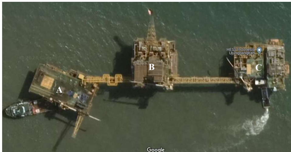
Gambar I.2 Fasilitas Offshore Production Facility SIPL
