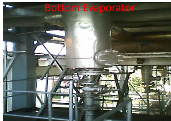
Gambar II. 5 Evaporator
