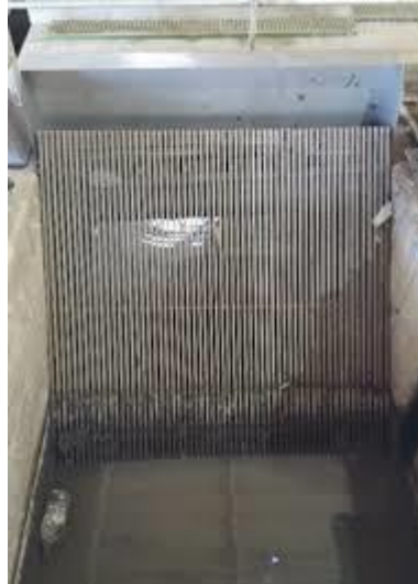
Gambar 2.3 Bar Screen Tipe Manual
