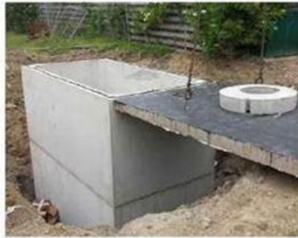
Gambar 2. 24 Reservoir Beton Cor
