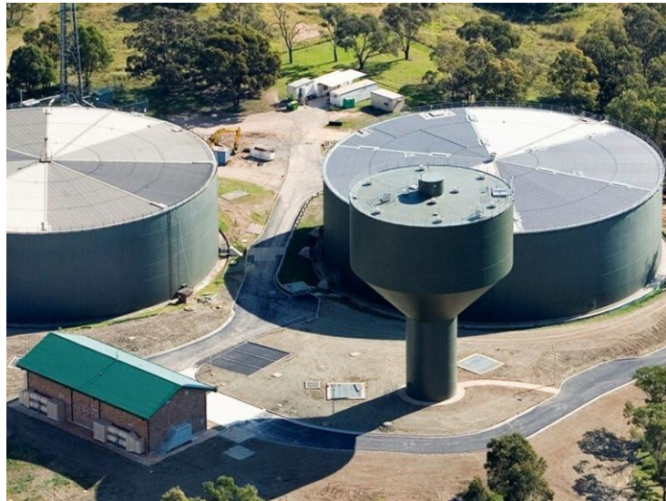
Gambar 2. 23 Reservoir Tangki Baja (Sumber: BPSDM PU, 2018)
