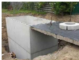
Gambar 2.14 Reservoir Beton Cor
