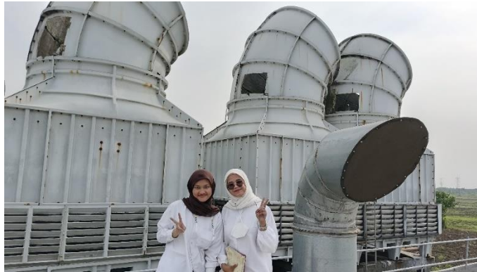
Gambar 2.6 Visit Cooling tower dan Reverse osmosis Perusahaan
