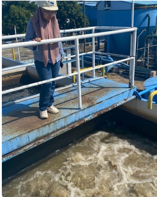
Gambar 2.10 Mengamati Proses Backwash Filter IPA 3
