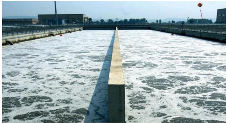
Gambar 2.8 Activated Sludge Contact Stabilization
