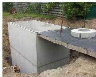
Gambar 2. 19 Reservoir Beton Cor
