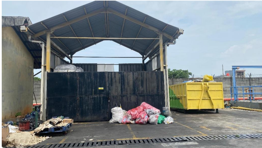
Gambar 2. 10 Kondisi TPS Eksisting PT Pertamina Lubricants
