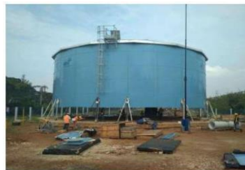
Gambar 2. 24 Reservoir Tangki Baja
