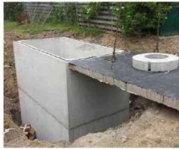
Gambar 2. 25 Reservoir Beton Cor
