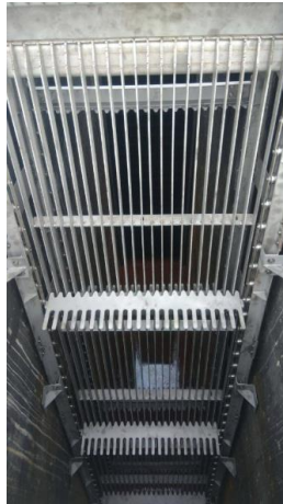
Gambar 2. 3 Coarse Screen / Penyaring Kasar
