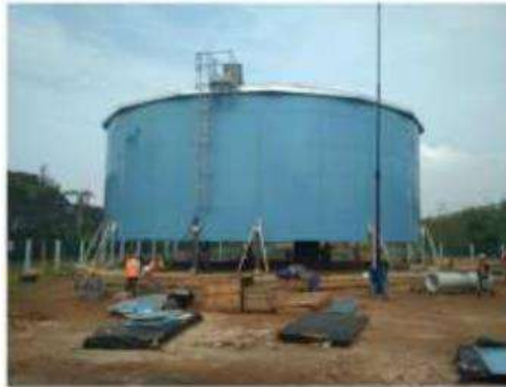
Gambar 2. 25 Reservoir Tangki Baja
