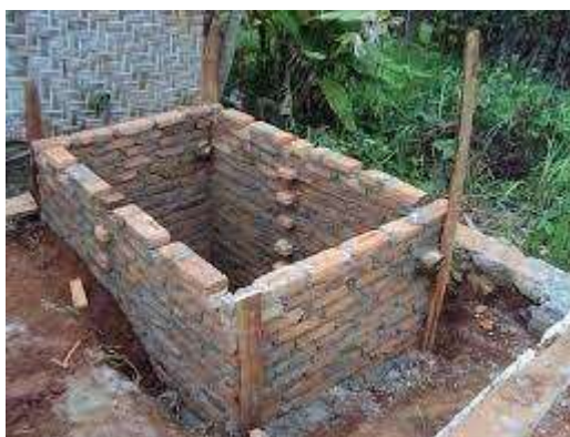
Gambar 2. 9 Reservoir Pasangan Bata
