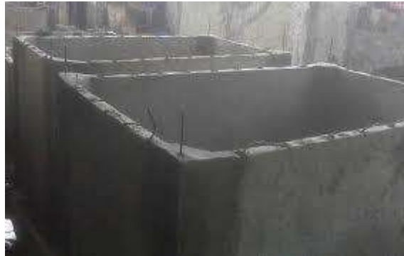
Gambar 2. 7 Reservoir Beton Cor
