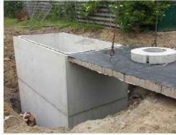
Gambar 2. 11 Reservoir Beton Cor
