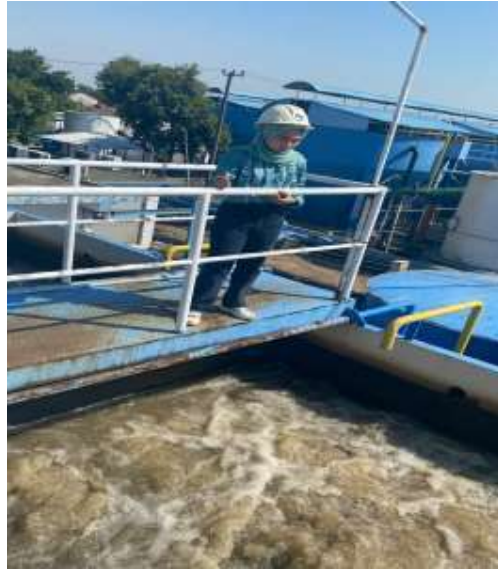
Gambar 2.7 Mengamati proses backwash
