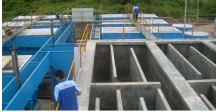
Gambar 2. 5 Bak Koagulasi-Flokulasi
