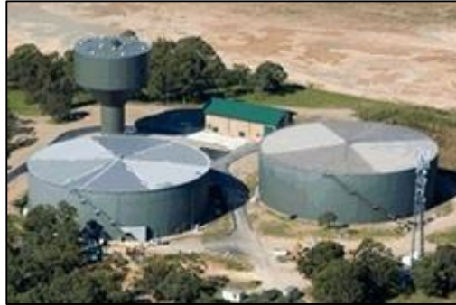
Gambar 2 15 Reservoir Tangki Baja
