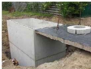
Gambar 2 16 Reservoir Beton Cor
