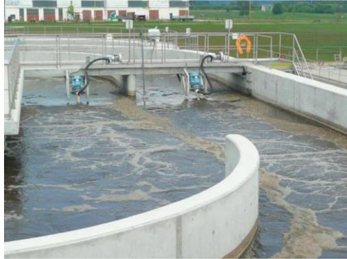
Gambar 2.12 Activated Sludge Oxidation Ditch
