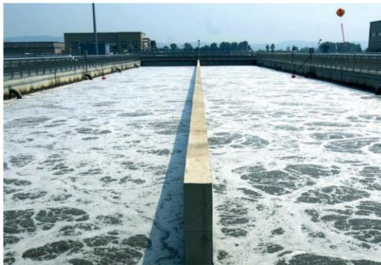
Gambar 2.8 Activated Sludge Contact Stabilization
