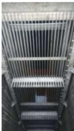
**Gambar 2. 3 Coarse Screen / Penyaring Kasar**
