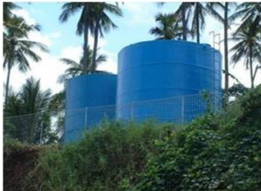
**Gambar 2. 26** Reservoir *Fiberglass*
