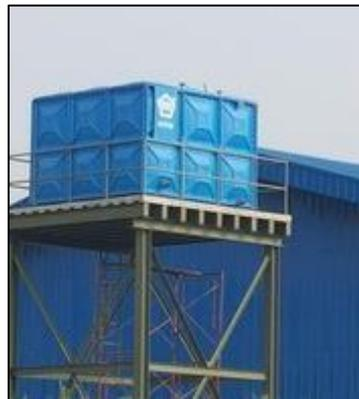
**Gambar 2. 25** Reservoir Fiberglass
