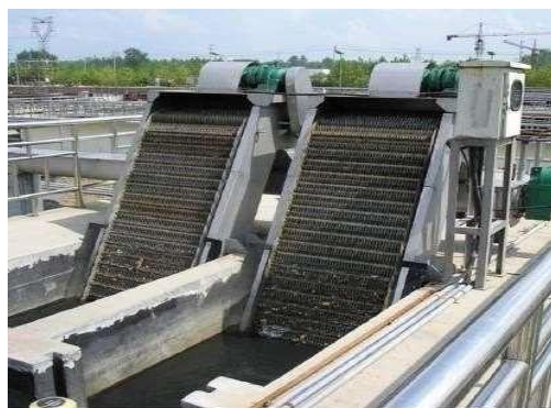
Gambar 2.3 Mechanical Bar screen
