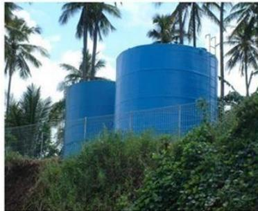
**Gambar 2. 31** *Reservoir Fiberglass*
