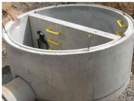
**Gambar 2. 30** Reservoir Beton Cor
