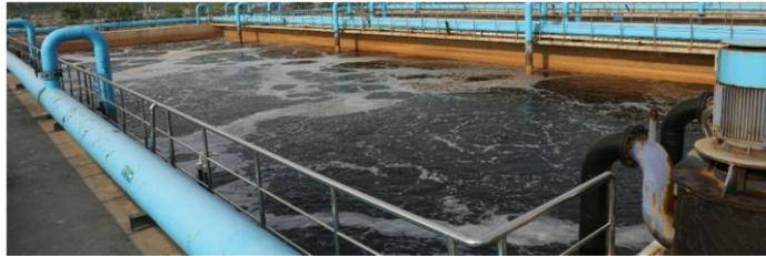
**Gambar 2.7** Activated Sludge
