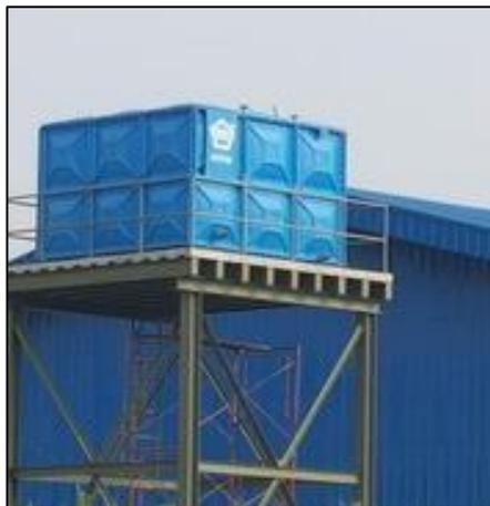
**Gambar 2.22** Reservoir *Fiberglass*
