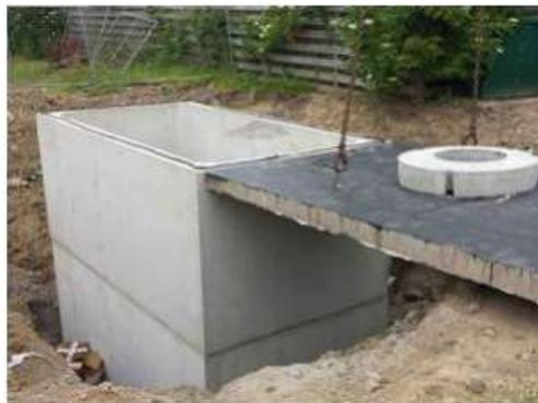
**Gambar 2. 14** Reservoir Beton Cor
