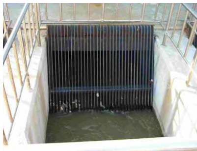
Gambar 2.5 Bar screen pembersihan manual
