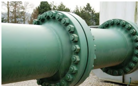
Gambar 2.35 Flange Pipa
