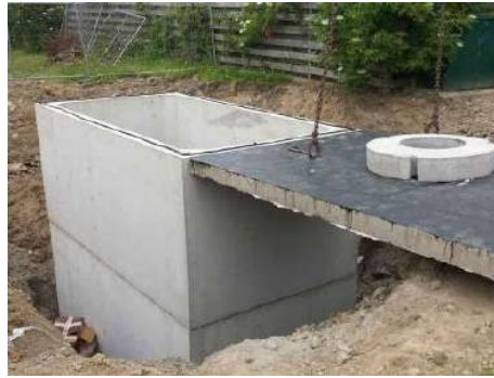
Gambar 2. 29 Reservoir Beton Cor
