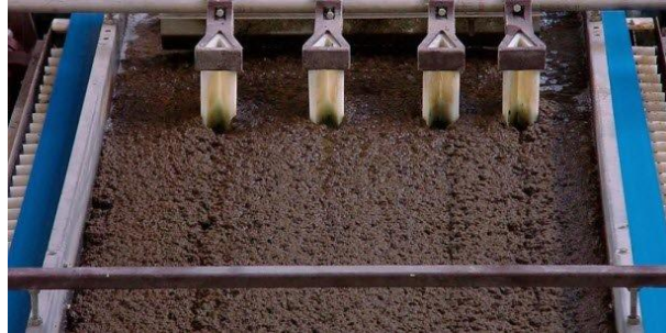
Gambar 2. 17 Sludge Drying Bed
