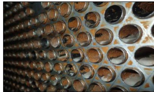
Gambar 2. Tube Brine Heater Setelah Cleaning
