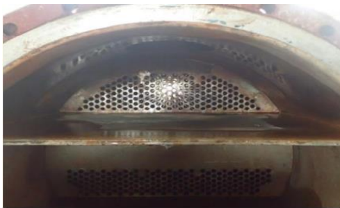
Gambar 17. Tube Condensate Cooler Setelah Cleaning
