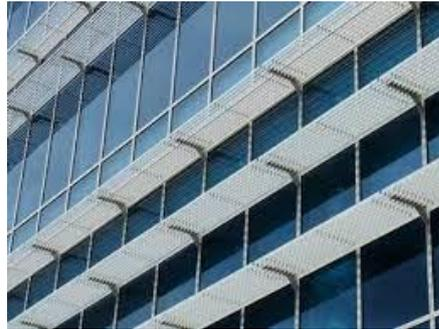
Gambar 5.18 Sun Shading
