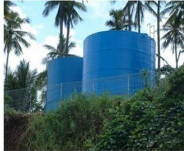
Gambar 2. 33 Reservoir Fiberglass
