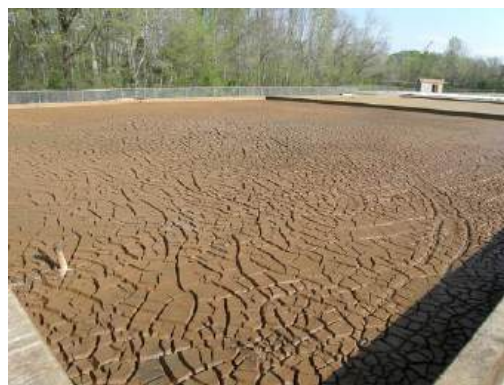
Gambar 2.25 Sludge Drying Bed
