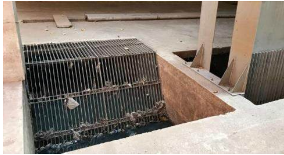
Gambar 2.3 Unit Bar screen
