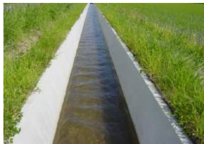
Gambar 2.1 Open Channel Flow
