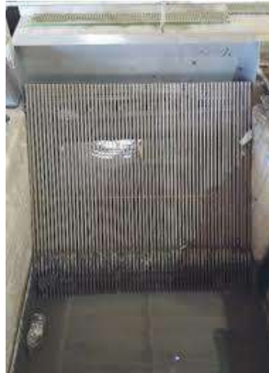
Gambar 2. 3 Bar Screen Tipe Manual
