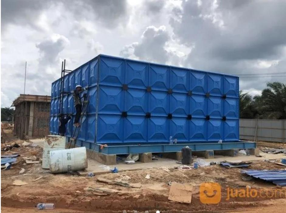
**Gambar 2. 33** *Reservoir Fiberglass*
