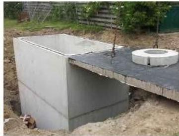
Gambar 2. 17 Reservoir Beton Cor
