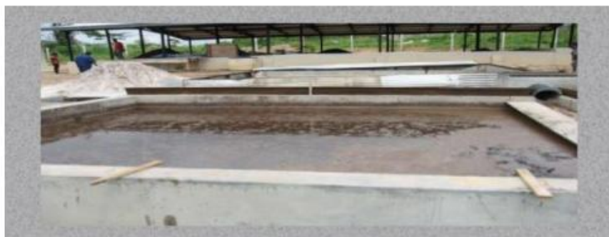
Gambar 2.22 Sludge Drying Bed
