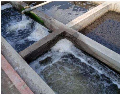
**Gambar 2. 7** Biofilter Aerob
